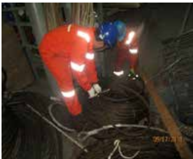
TOWING WIRE PREPARATION
