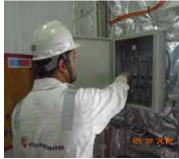
VENT TEAM CLOSING ACCOMMODATION FANS
